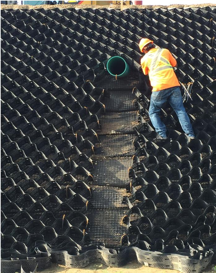
Geo-cell cut in order to make channel for CC
