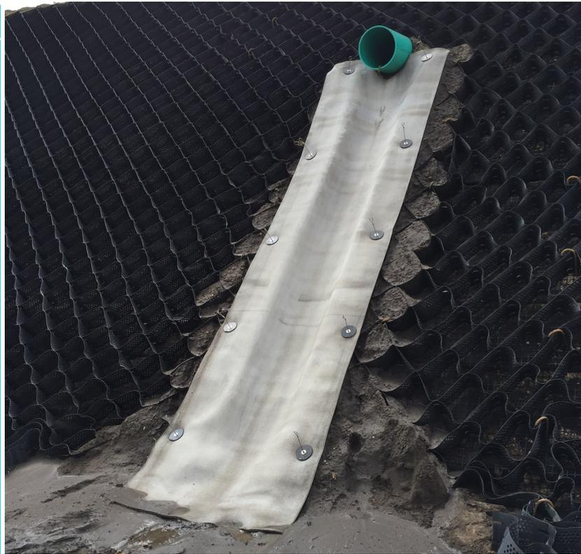
In July of 2016, 50 sq. m of Concrete Canvas 8mm (CC8) was used to line 8 outfalls on the side slope of a roadway in Saskatoon, SK, Canada. Each outfall was approximately 1m wide and 6 m long.
