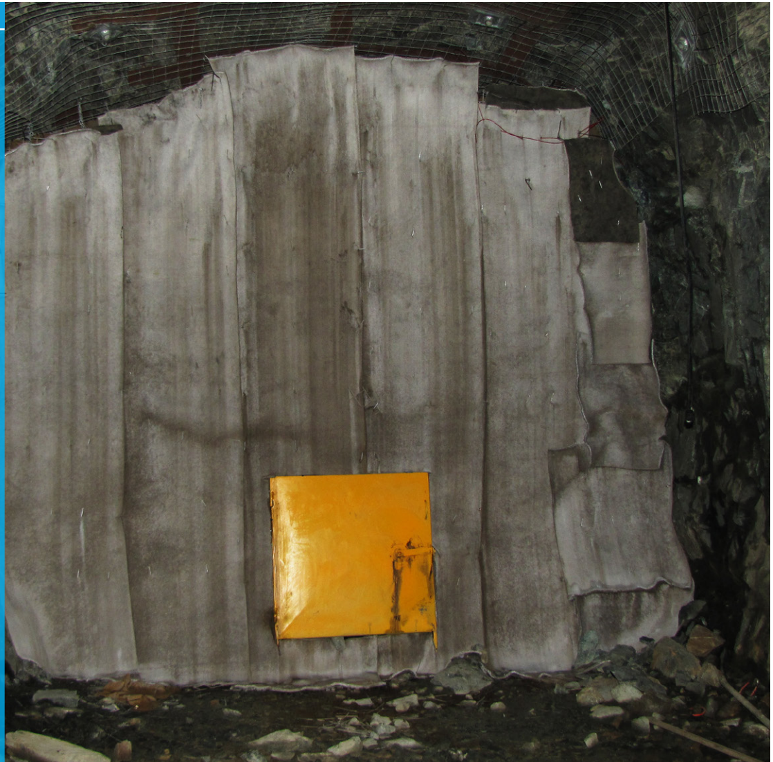
Finished vent wall
