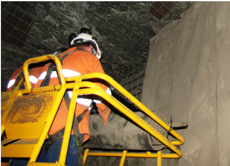
CC loaded onto elevated work platform
