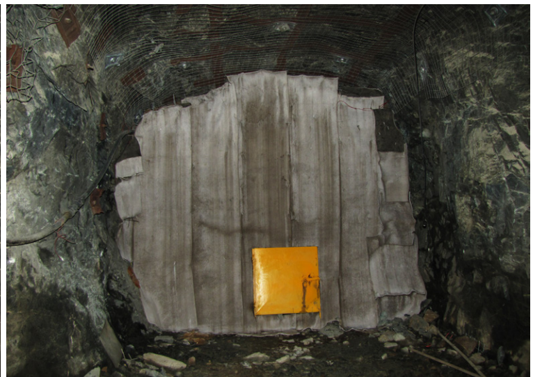
Finished vent wall installation
