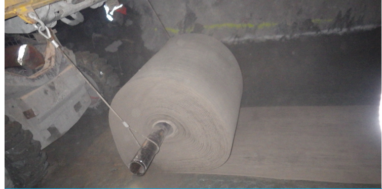
Concrete Canvas installarion
