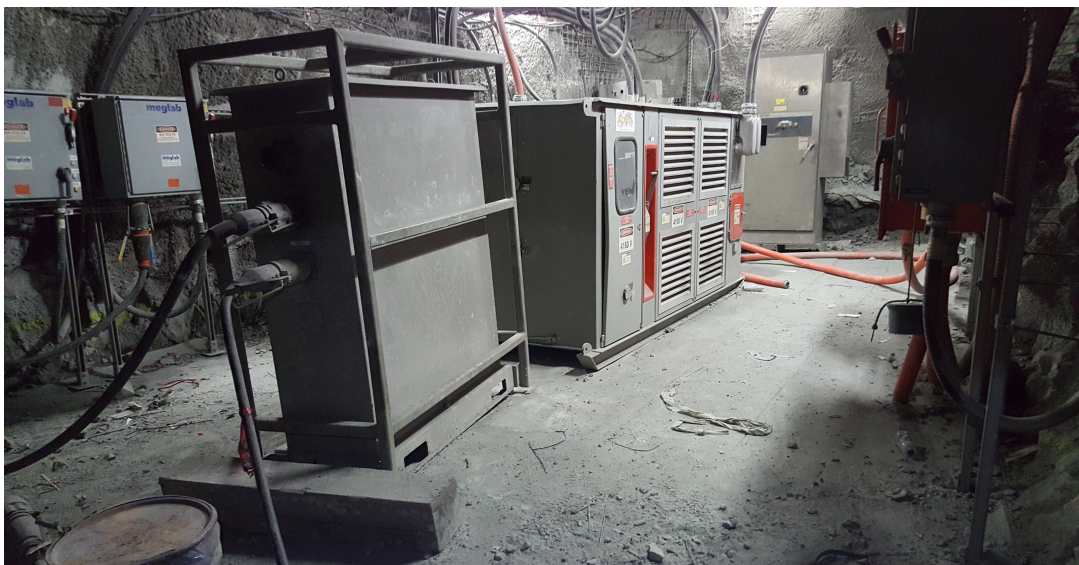
Installation 6 months later
